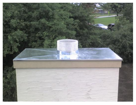
For those with prefabricated or factory-built chimneys, a <u>chase cover</u>, or chase top, is what's found on top covering the opening of your chimney. It does the same job as a chimney crown on a masonry chimney.
