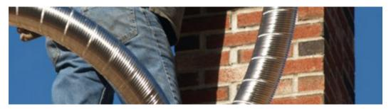
Another chimney part that's absolutely essential to your home's safety is the chimney liner. Chimney liners encase the walls of your chimney and lead smoke up and out of it.
