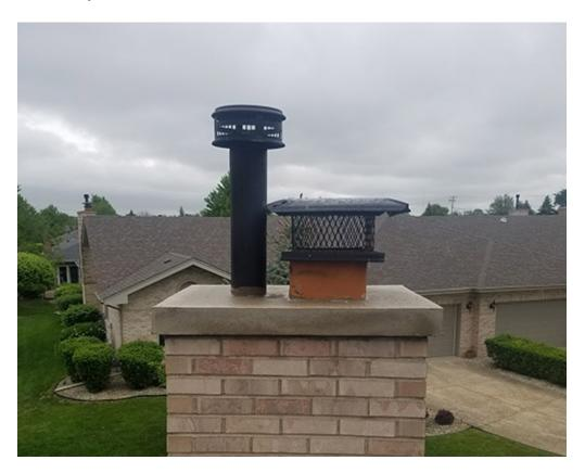
Not to be confused with chimney caps, chimney crowns are also on top of the chimney. However, they're only found on masonry chimneys and not prefabricated or factory-built ones.
