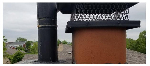
Chimney caps are found on the top of the chimney and protect against rain, snow, debris and even animals from getting into your chimney.
