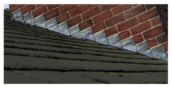
Flashing is found where your chimney meets the roof. It helps protect your chimney from moisture penetration. Chimney flashing can be made of aluminum, steel, copper or vinyl and it's crucial to have flashing that's in good condition.
